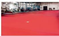
Anti-microbial floor & wall systems provide superior protection against bacterial and microbial growth. These systems provide a hygienic barrier by penetrating into the concrete substrate.
