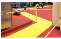
Food grade safety coatings are available to communicate traffic patterns or OSHA 5-S safety protocols. Safety coatings provide resistance to chemicals and wet environments.
