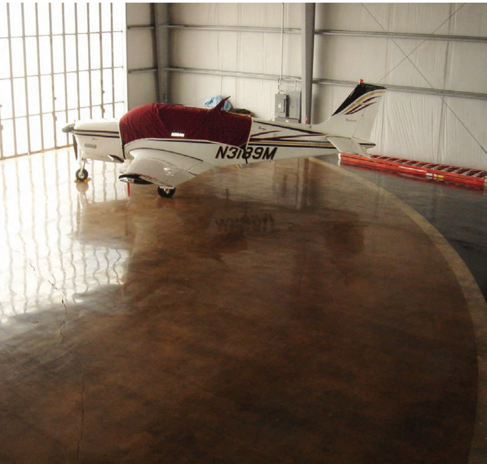
Level C, Heavy Aggregate, Dye, Airplane Hangar, 5+ Years Old
