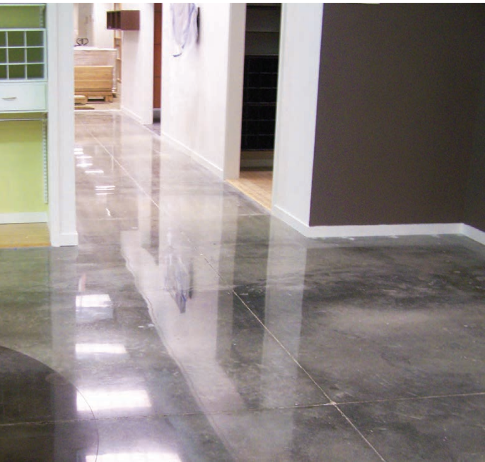
Level C, Medium to Heavy Aggregate, Natural & Stain, Office
