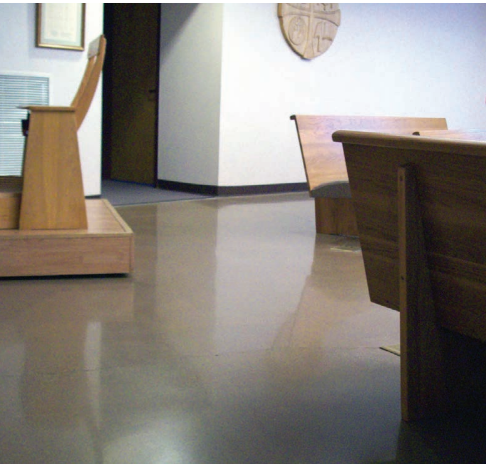
Level B, Medium Aggregate, Integral Color, Church, 8 Years Old
