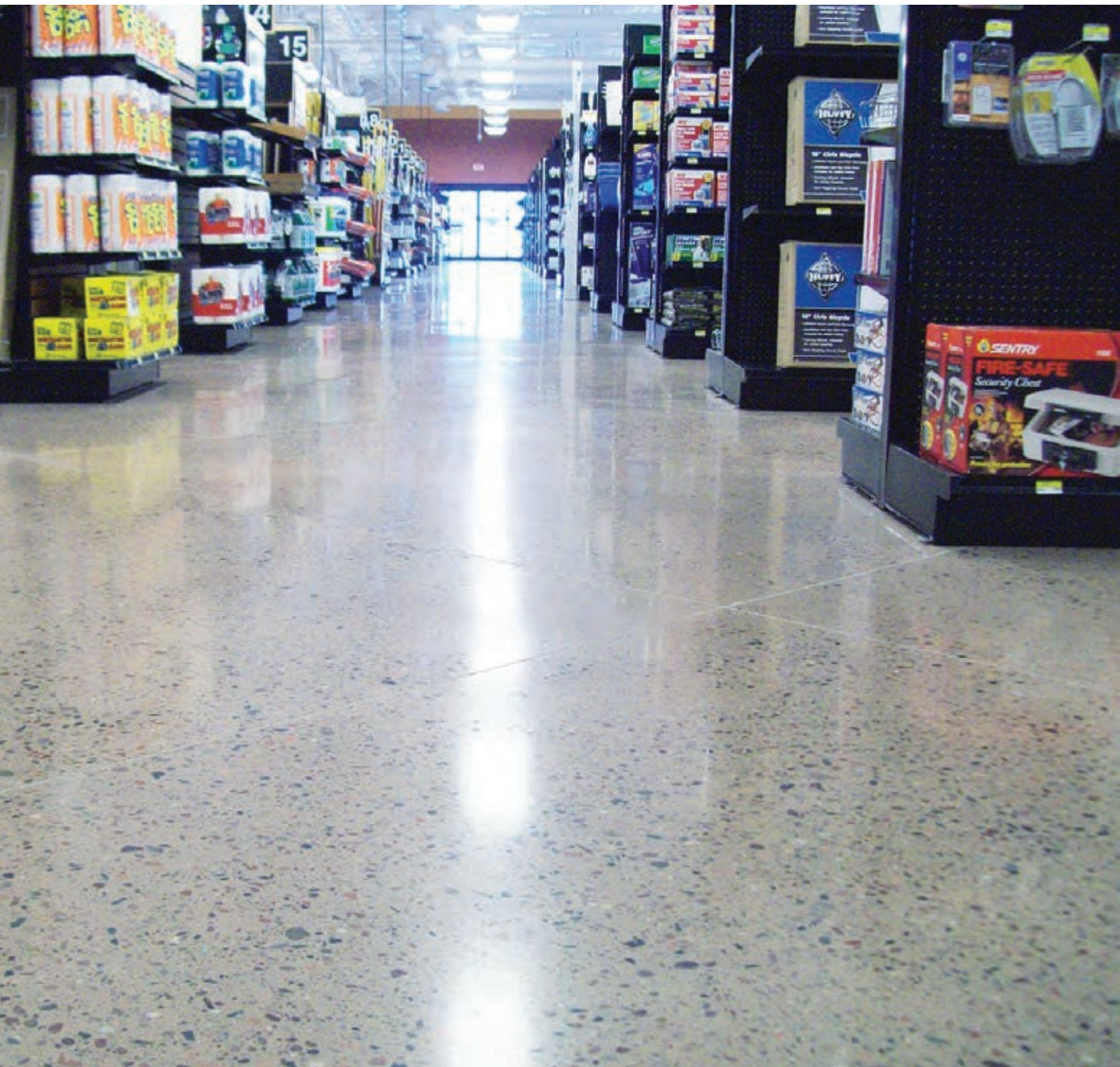
Level B, Heavy Aggregate, Natural Color, Hardware Store, 3 Years Old
