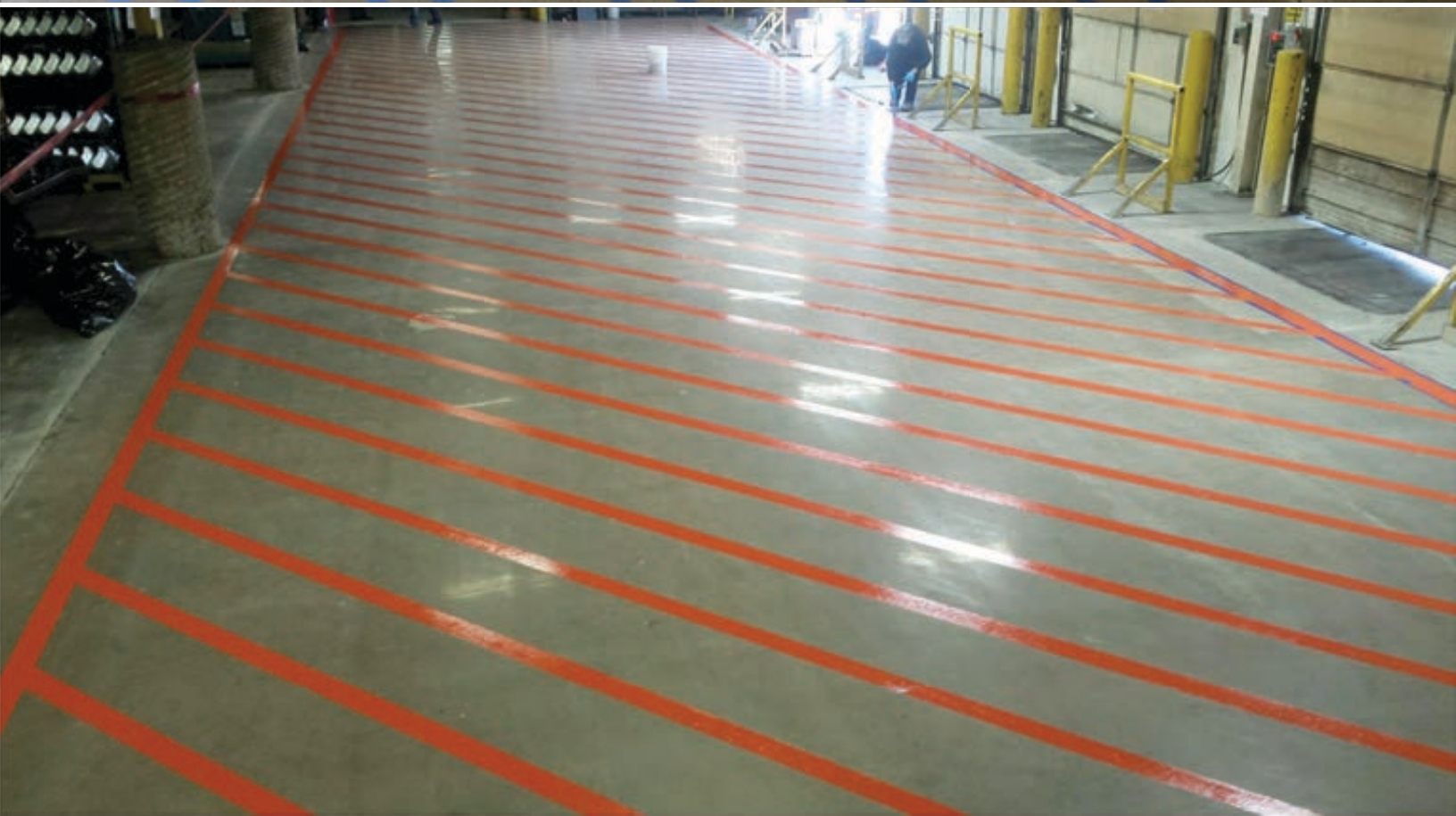
Polished Concrete With Line Striping
