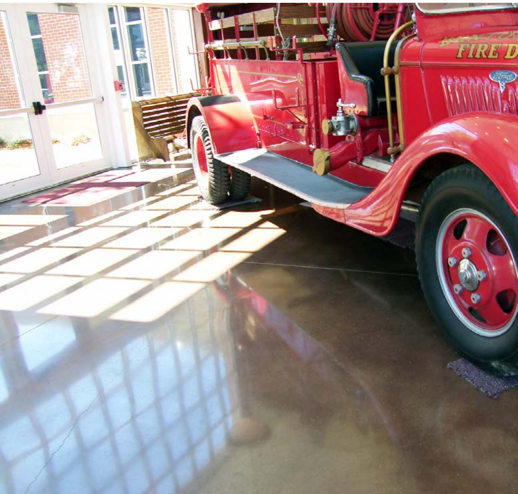
Level B, Medium Aggregate, Natural Color, Fire Station
