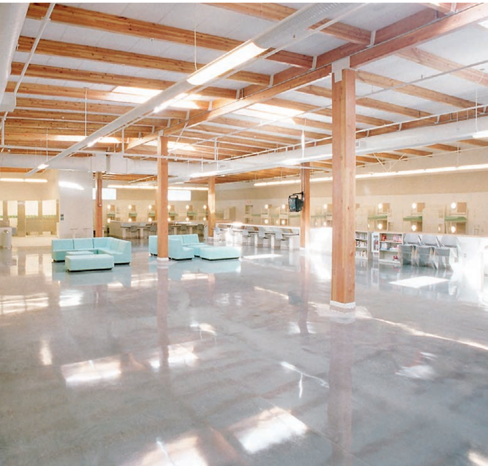
Level B, Light Aggregate, Natural Color, Correctional Facility, 5+ Years Old
