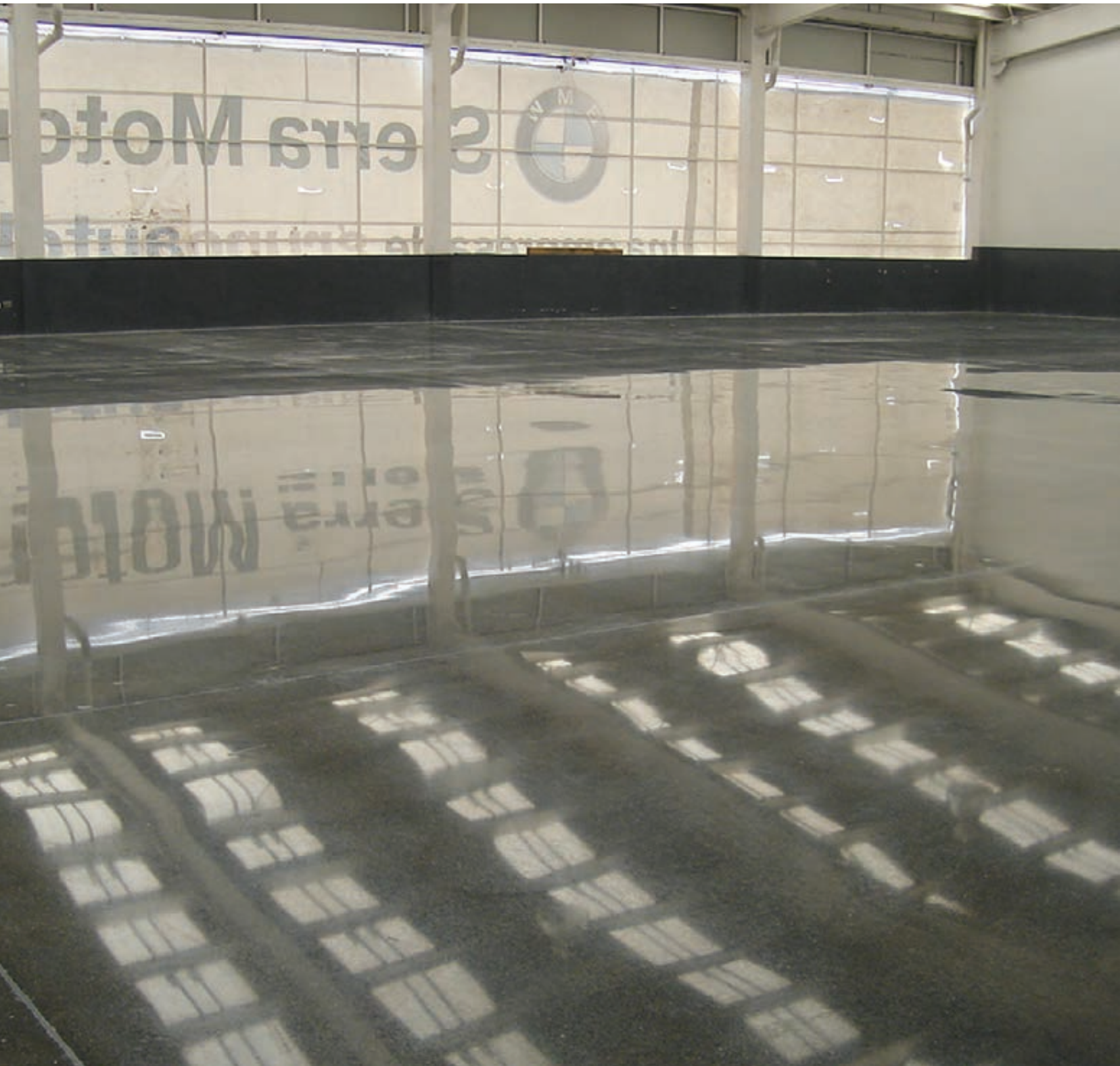
Level C, Light Aggregate, Colored, Manufacturing, 3+ Years Old
